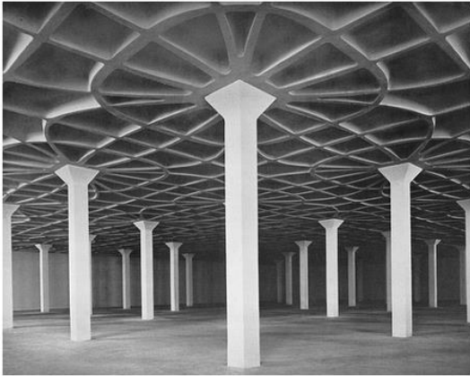
Pier Luigi Nervi Gatti Wool Factory Floor System (1953) https://en.wikipedia.org/wiki/Pier_Luigi_Nervi
