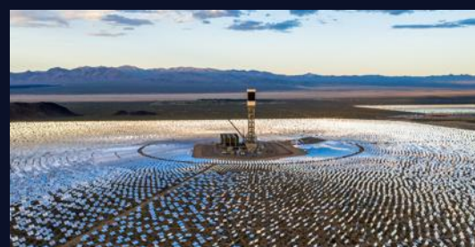
Concentrated Solar Power (CSP)
